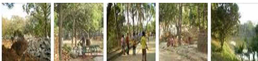
Internal Views of Shahid Matiur Park, People Moving around, Playing and Working in the Park, Construction Materials are Seen in the Photographs
